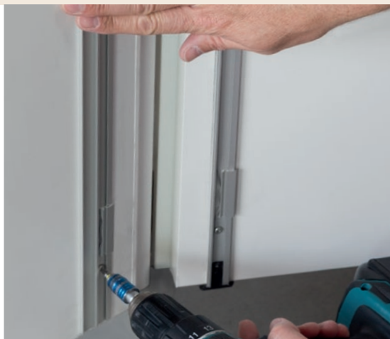
* 1. Building phase – only fixing profiles mounted
